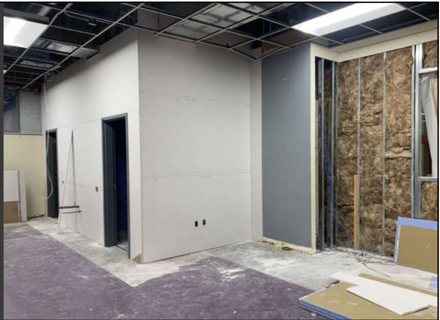
Restroom walls – insulated and closed in!
